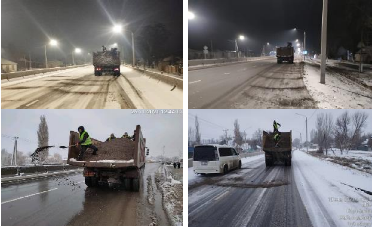
Figure 28 Sand sprinkling on the road. Control of ice
