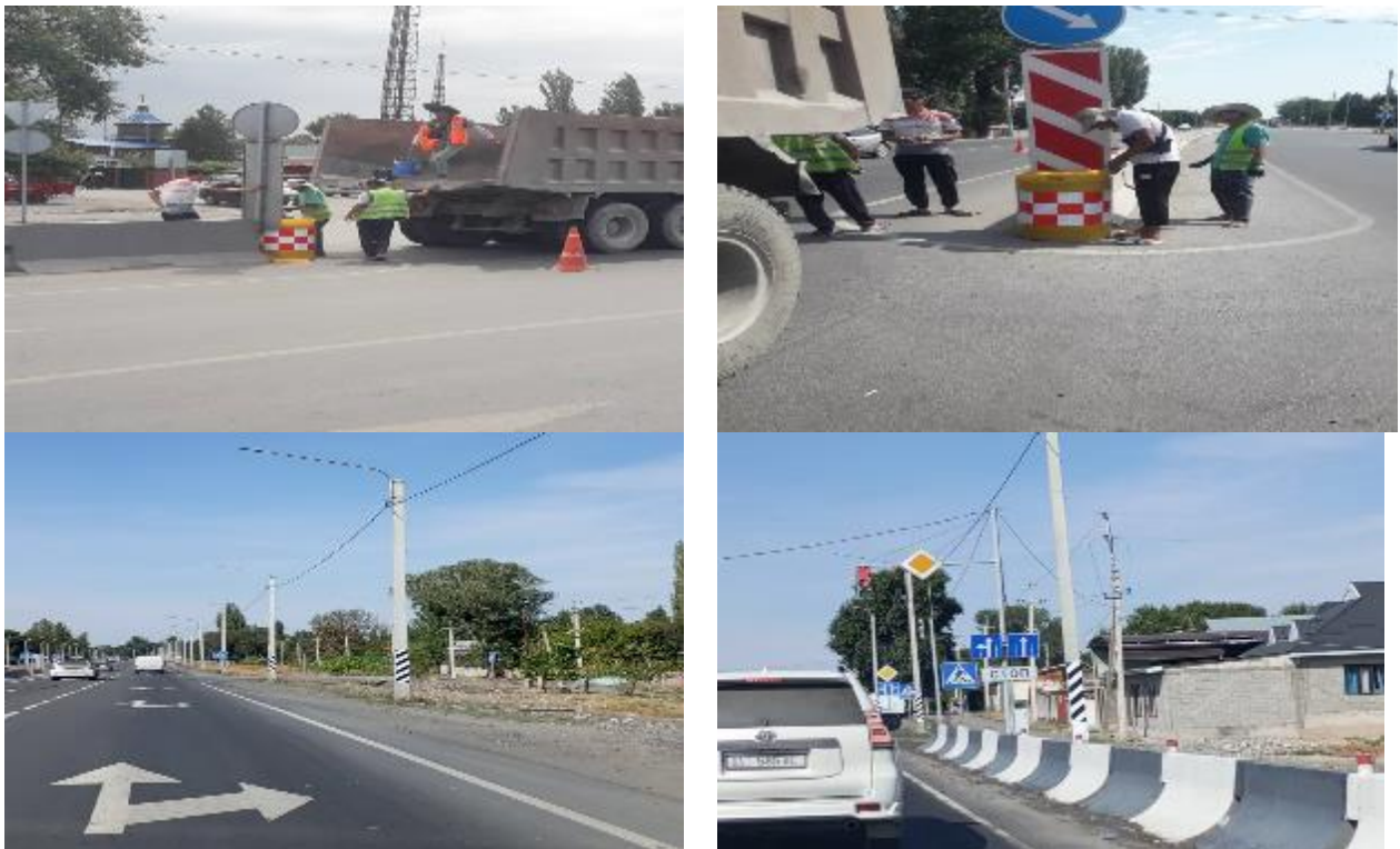
Figure 35 Installation of anti shock buffers. Application of road marking
