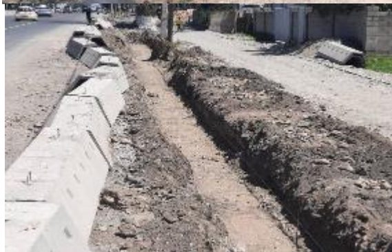
Figure 26 Construction of drainage ditches and OP- 1 slabs above the ditch
