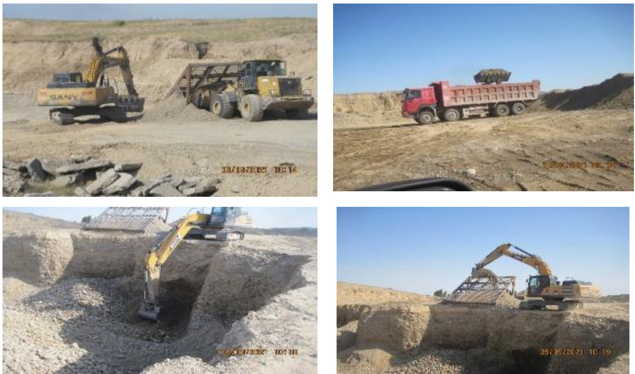
Figure 11 Development of Belek borrow pit
