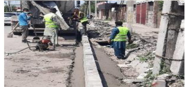
Figure 31 Installation of curbs
