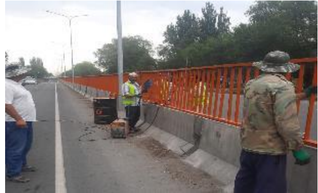
Figure 20 Installation of metal guardrails
