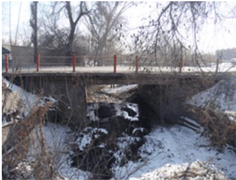
Figure 22 Discharge canal in the village of Novopavlovka
