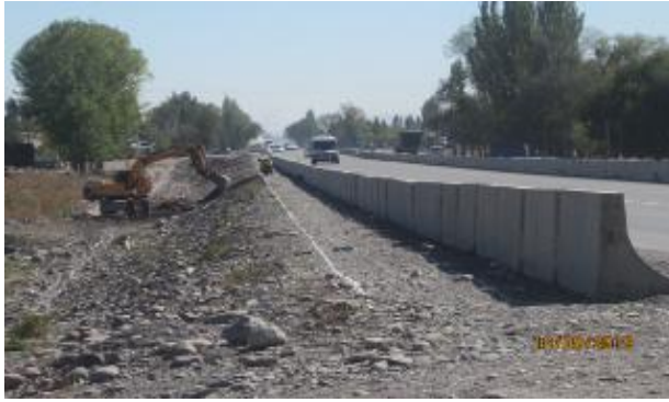
Figure 29 Installation of "Sapojok" type parapets.
