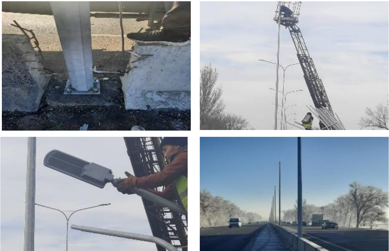
Figure 36 Foundation of street lighting poles and installation of metal poles
