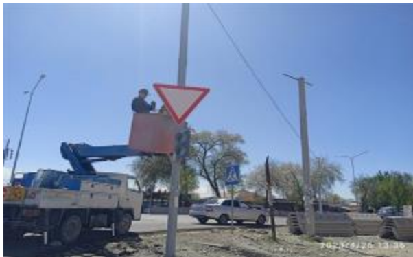
Figure 18 Installation of road signs
