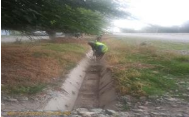
Figure 30 Cleaning drainage ditches
