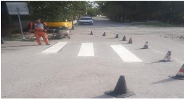
Figure 19 Application of road marking
