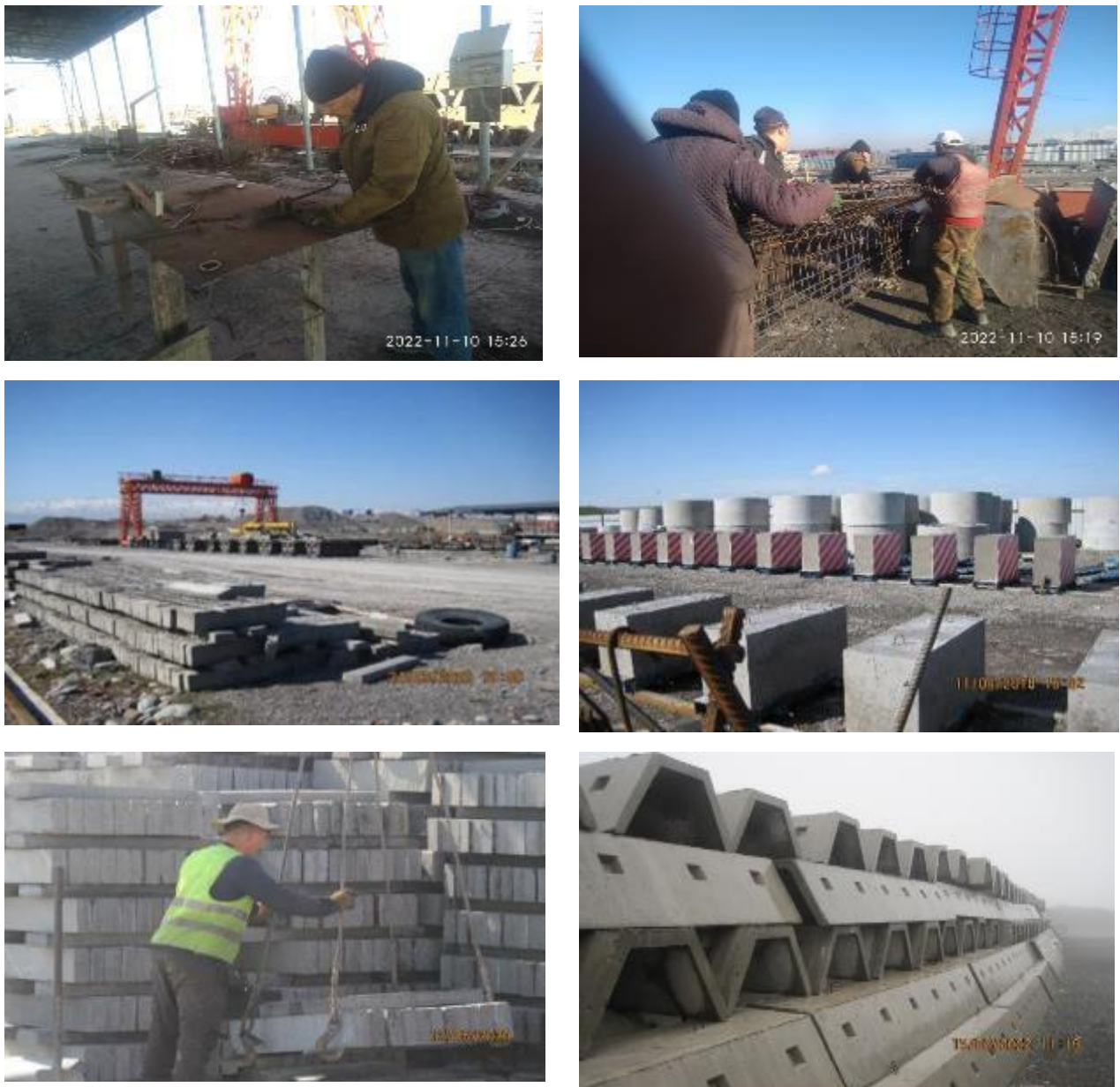
Figure 39 Manufacture and preparation of reinforced concrete structures
