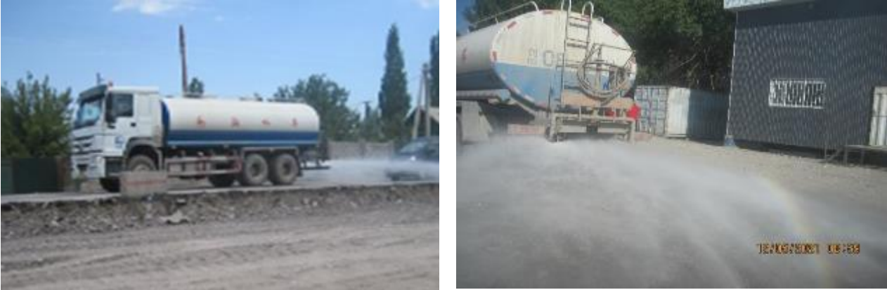
Figure 20 Dust suppression works (water sprinkling) on construction sites
