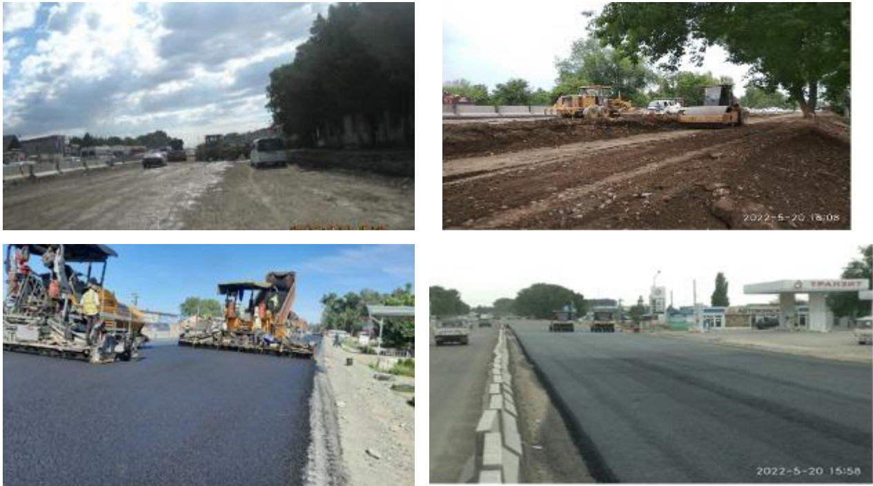
Figure 18 Rolling, compaction of soil and asphalt paving of the carriageway
