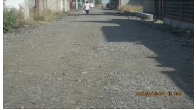
Figure 53 Streets backfilled with old asphalt
