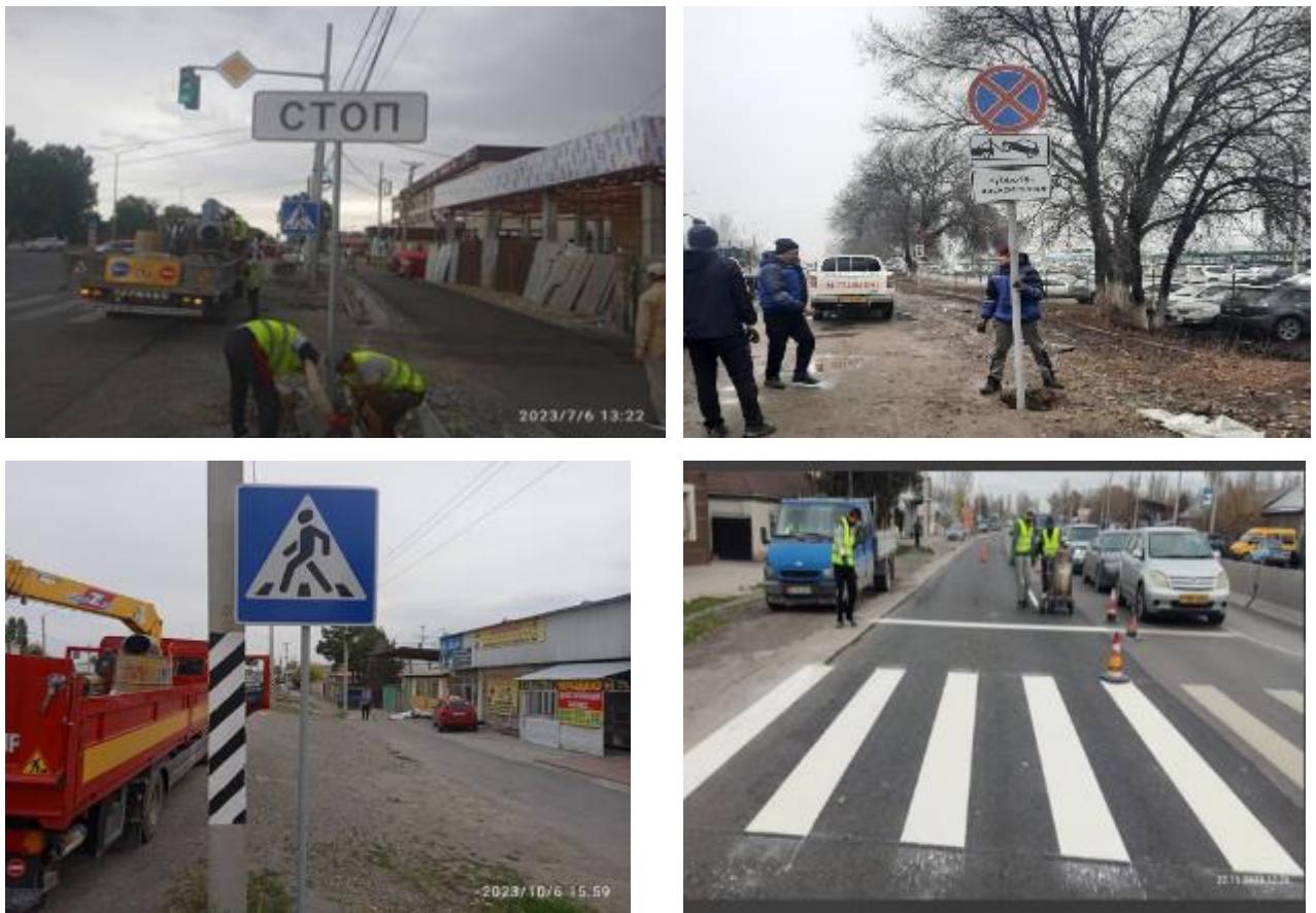
Figure 52 Installation of road signs and application of road marking
