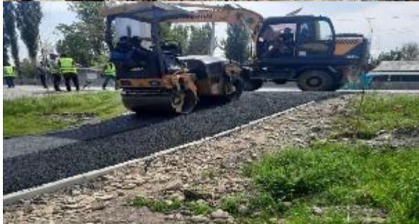
Figure 6 Construction of jointing walkways
