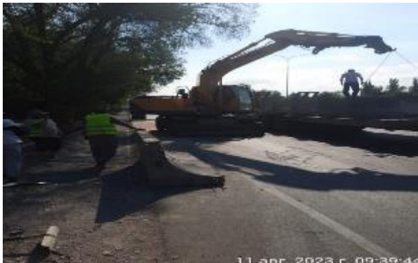
Figure 21 Installation of “Sapojok” type parapets
