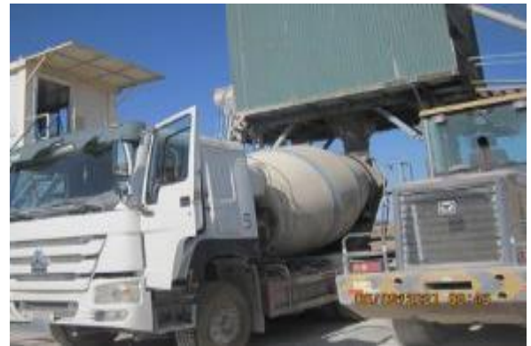
Figure 43 Filling the concrete mixing machine with concrete
