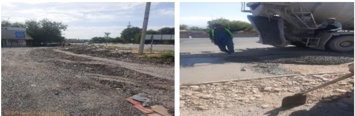
Figure 4 Construction of sidewalks
