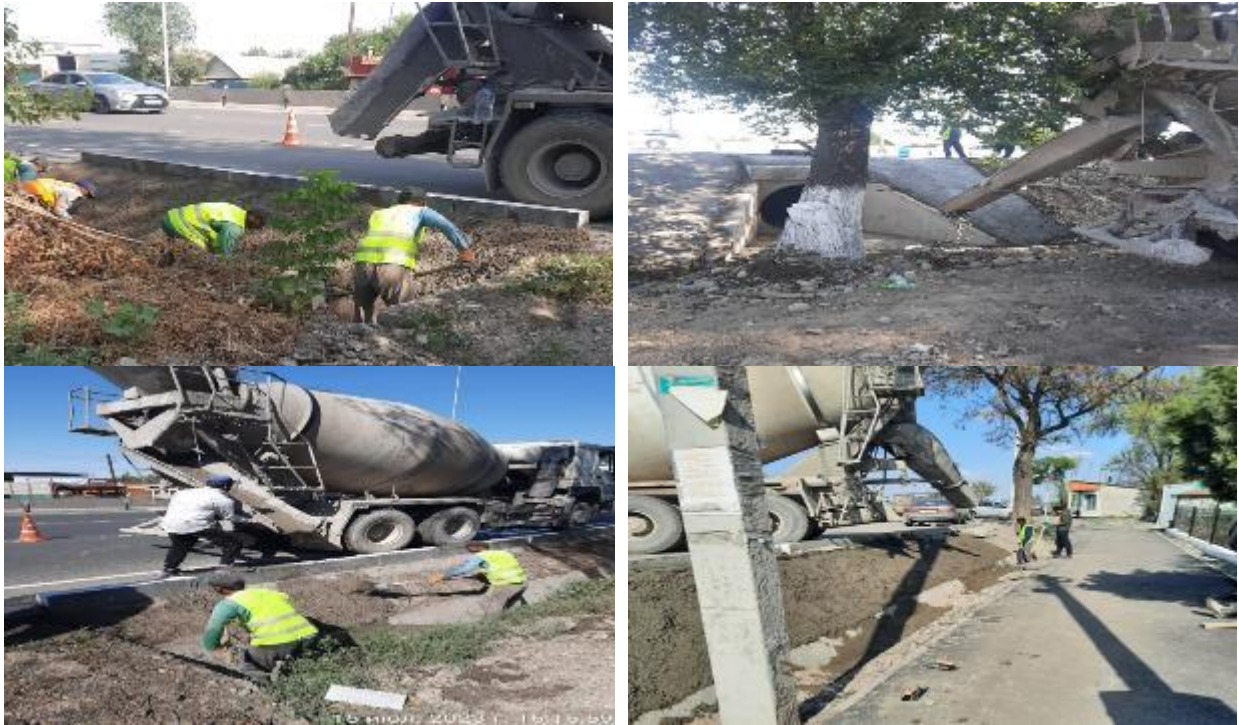
Figure 15 Cleaning and strengthening of shoulders
