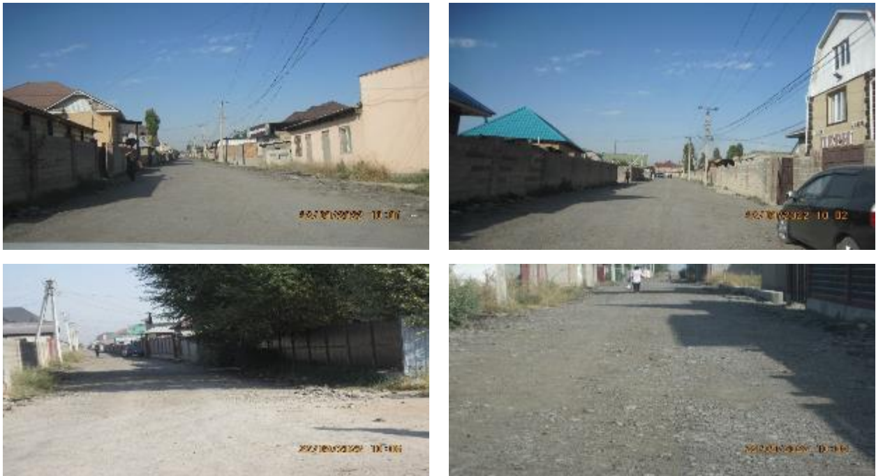
Figure 45 Streets paved with old asphalt at 7.4 km section
