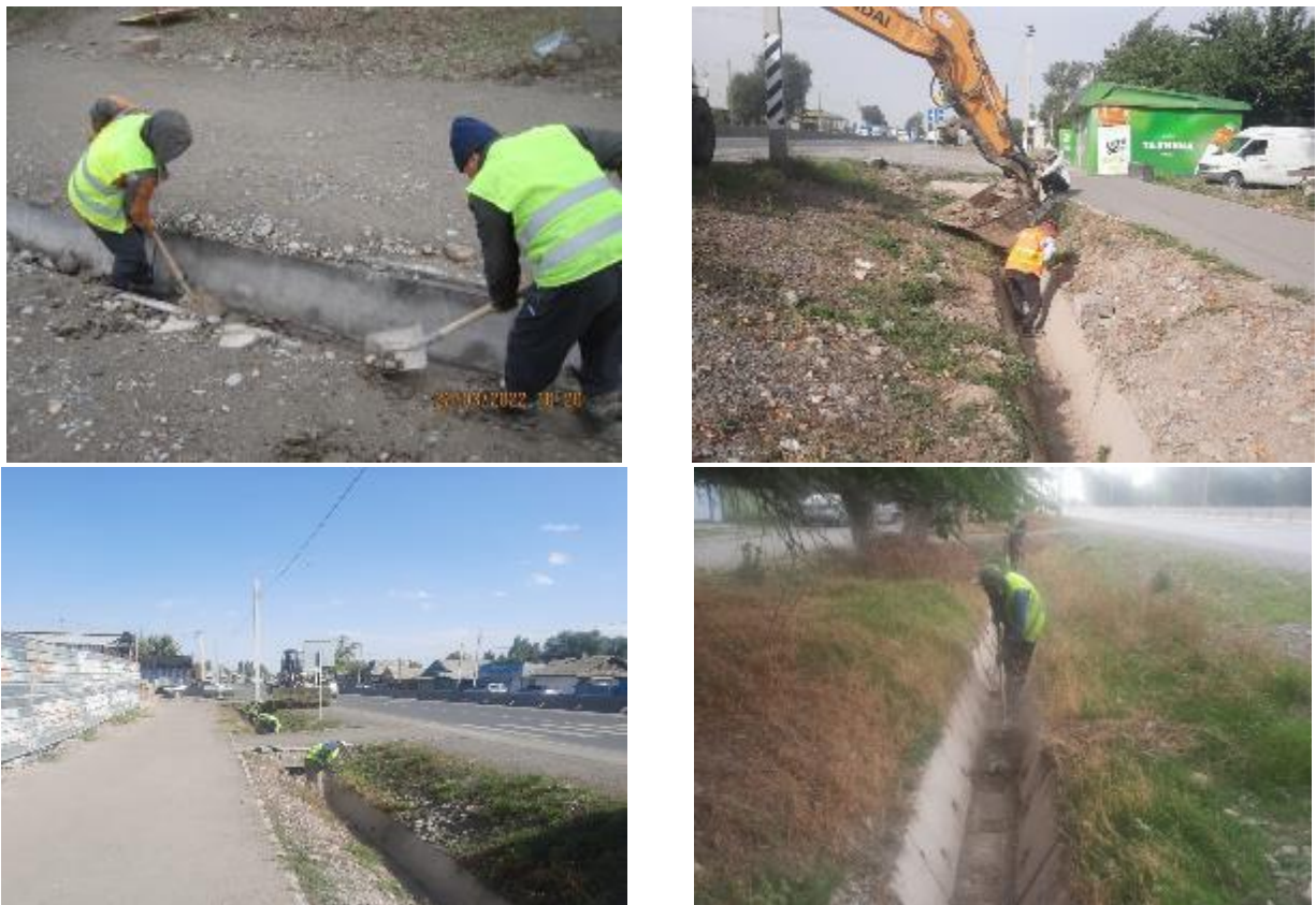
Figure 27 Cleaning of drainage ditches
