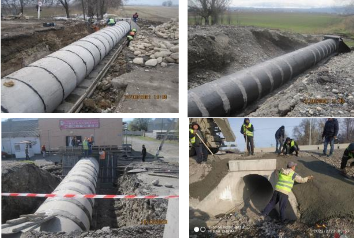
Figure 24 Construction of culvert pipes
