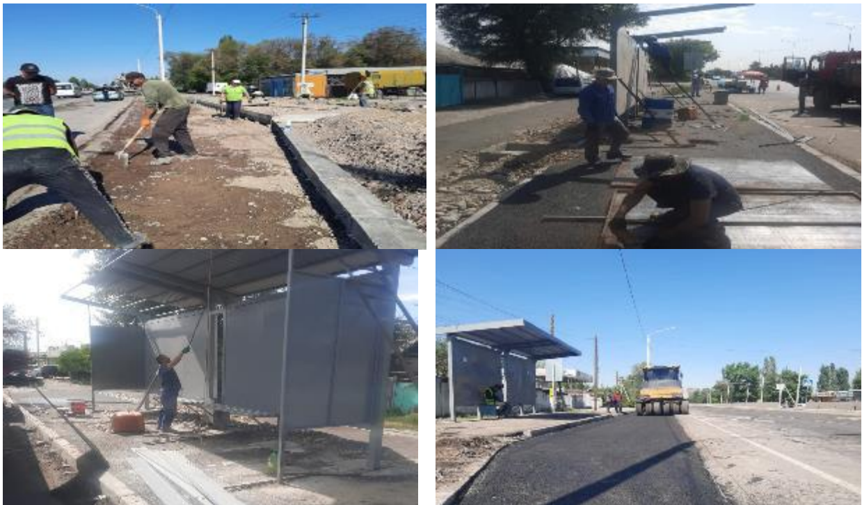
Figure 16 Construction of bus stops and paving area around it
