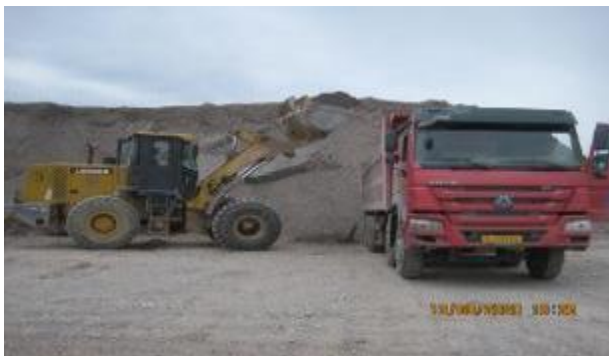
Figure 14 Development of Ak-Suu 2 borrow pit on moistened material
