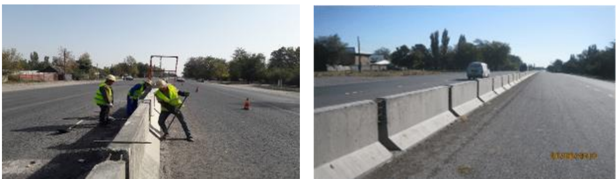
Figure 28 Installation of New Jersey type barriers
