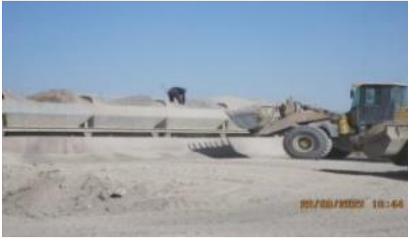
Figure 42 Preparation of gravel material for the production of concrete and asphalt
