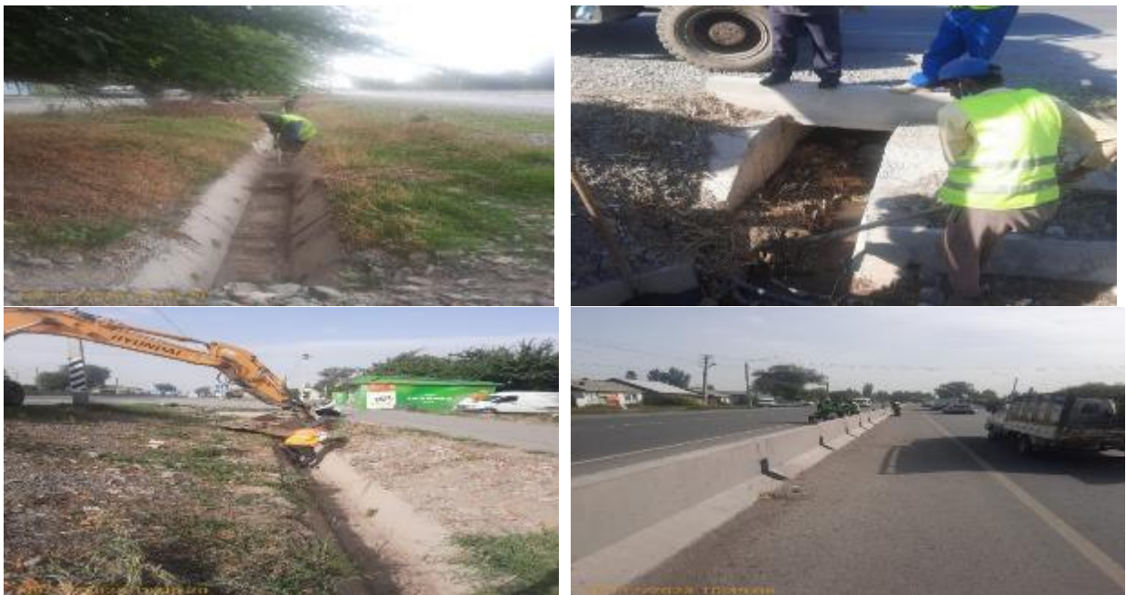
Figure 12 Removing debris on drainage ditches and parapets
