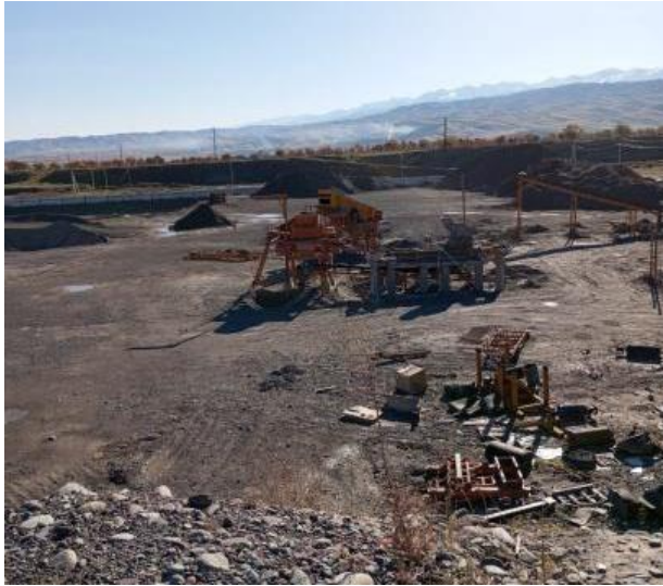
Рисунок 48 Dismantling of equipment on the production site
