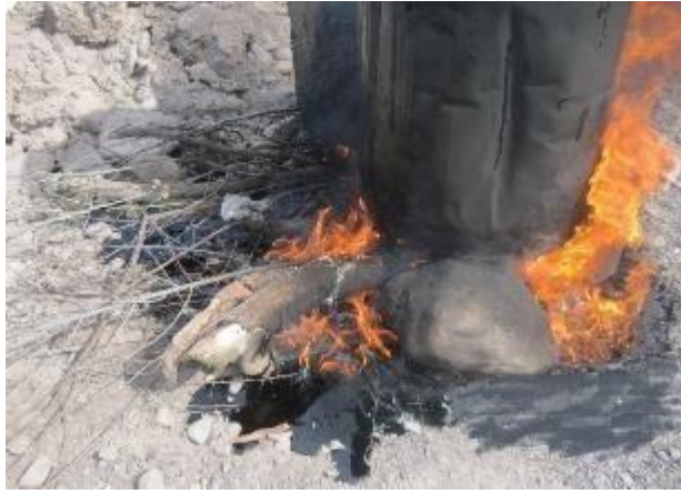
Figure 25 Bitumen melting for waterproofing of pipe
