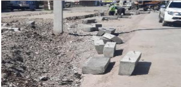
Figure 31 Installation of curbs
