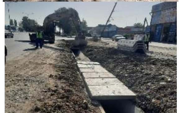
Figure 26 Construction of drainage ditches and OP- 1 slabs above the ditch
