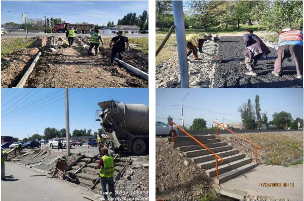
Figure 32 Construction of jointing walkways
