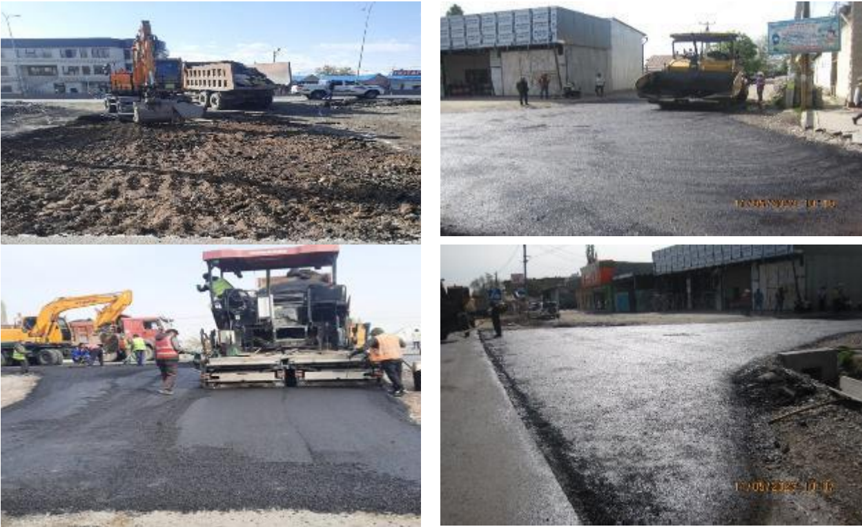
Figure 19 Construction of junctions to adjacent streets
