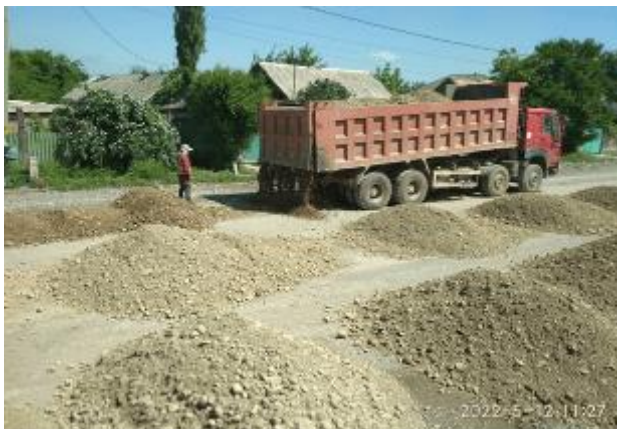
Figure 17 Levelling of roadbed in the village of Voенno-Antonovka
