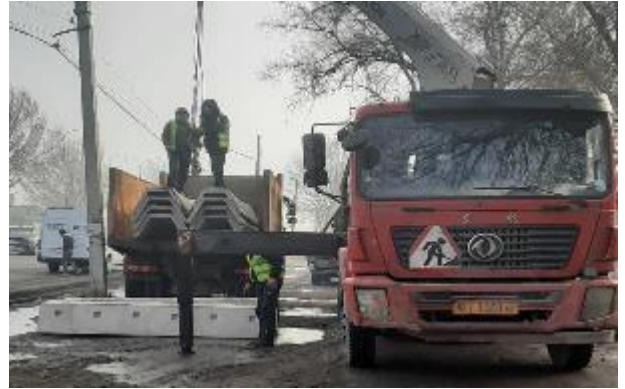
Figure 51 Failure to comply with safety precautions when moving load with a crane
