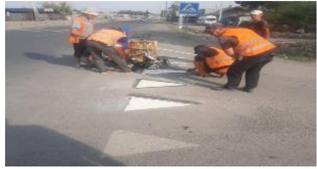
Figure 19 Application of road marking
