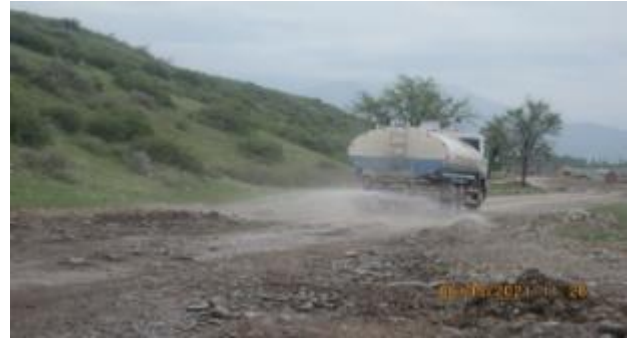
Figure 15 Water sprinkling on the access road to Ak-Suu 2 borrow pit
