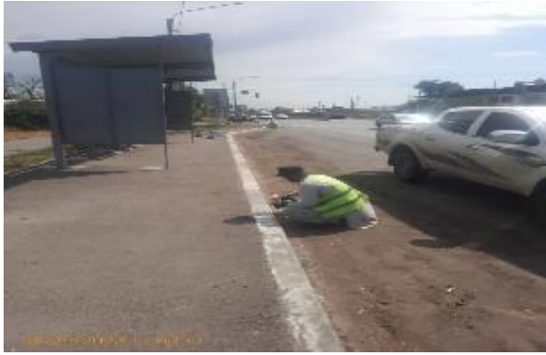
Figure 8 Installation of curbstones at bus stop areas
