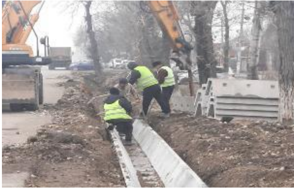
Figure 51 Failure to comply with safety precautions when moving load with a crane
