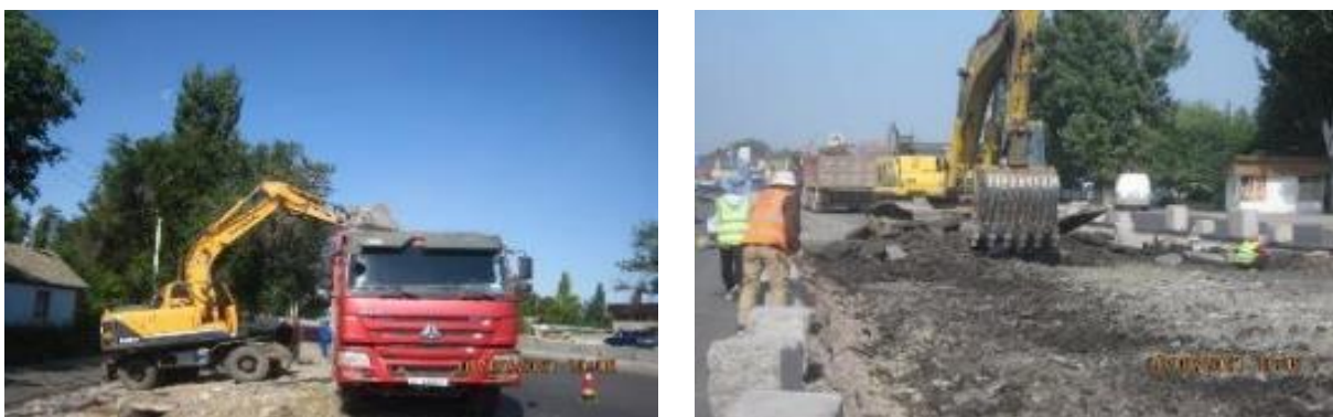
Figure 52 Taking out of removed asphalt in the Voенно-Antonovka village
