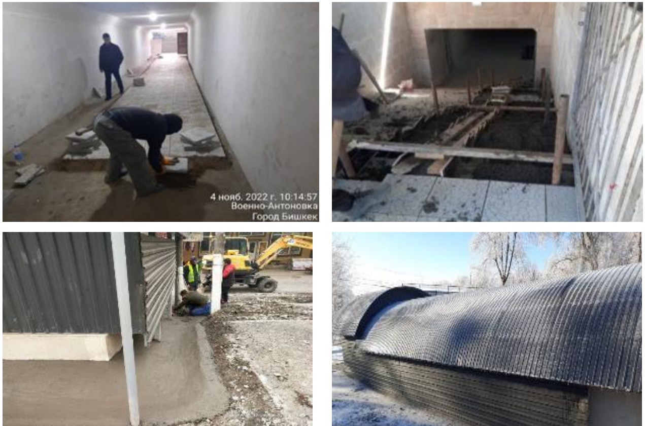
Figure 32 Construction works at the underpasses
