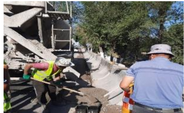
Figure 21 Installation of “Sapojok” type parapets
