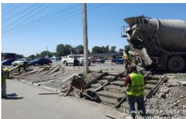
Figure 7 Construction of jointing walkways with steps
