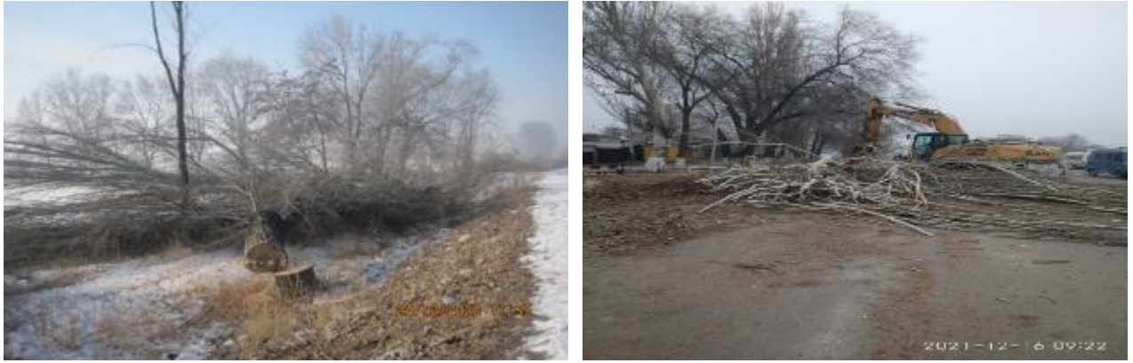
Figure 4 Tree cutting at km 8,5 – km 15,9 section
