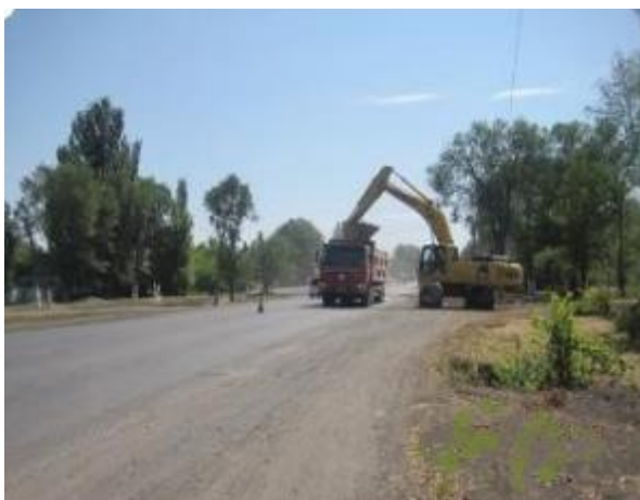
Figure 9 Removal of topsoil with water sprinkling
