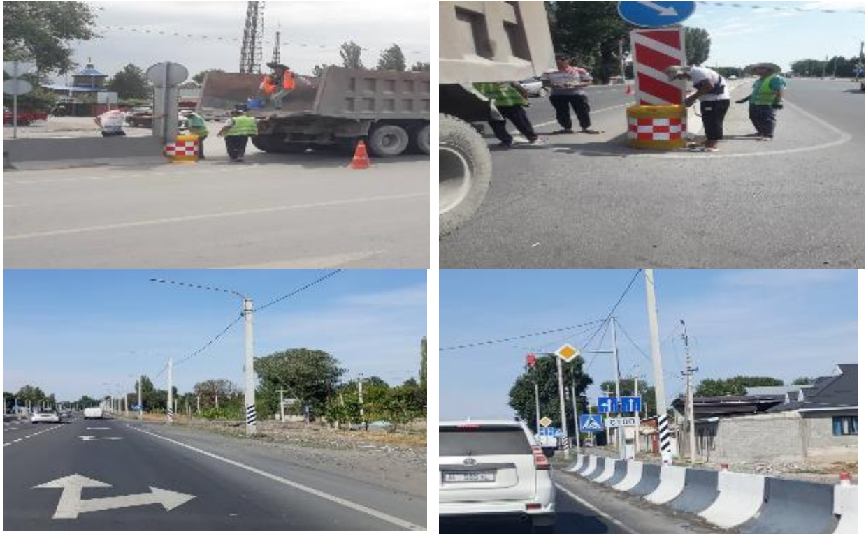
Figure 11 Installation of anti shock buffers. Application of road marking
