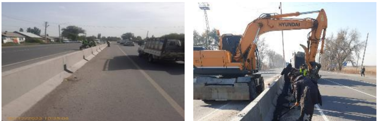
Figure 29 Cleaning and removal soil waste near parapets
