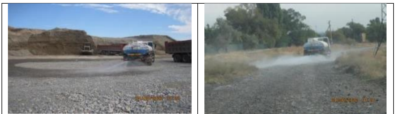
Figure 12 Water sprinkling on the access road to the Belek borrow pit
