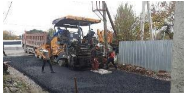
Figure 45 Loading of asphalt mixture into dump trucks and unloading into asphalt pavers
