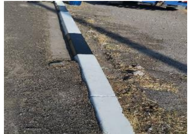
Figure 9 Painting parapets and curbstones
