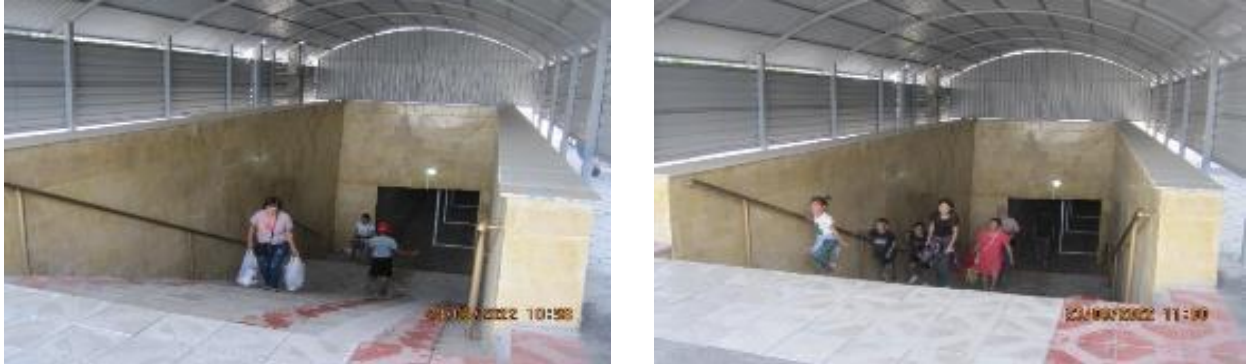
Figure 34 Underpass in the Sokuluk village
