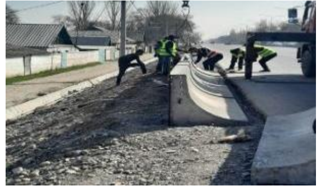
Figure 29 Installation of "Sapojok" type parapets.
