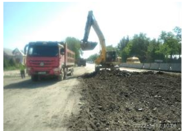
Figure 17 Levelling of roadbed in the village of Voенno-Antonovka
