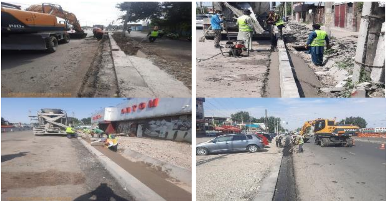
Figure 14 Installation of curbstone
