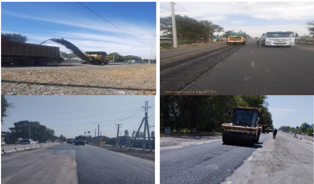
Figure 3 Milling and laying wearing course, removing rutting
