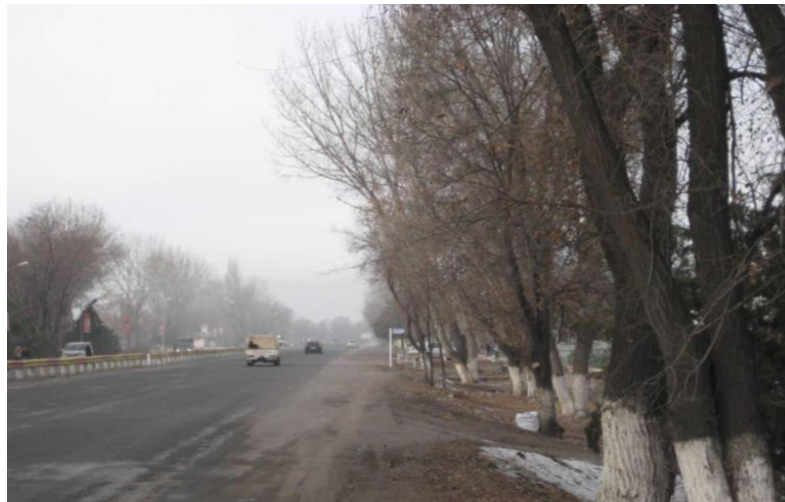
Figure 3 Road section before cutting down trees
