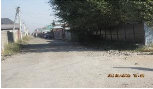
Figure 53 Streets backfilled with old asphalt
