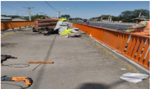
Figure 10 Installation of metal guardrails
