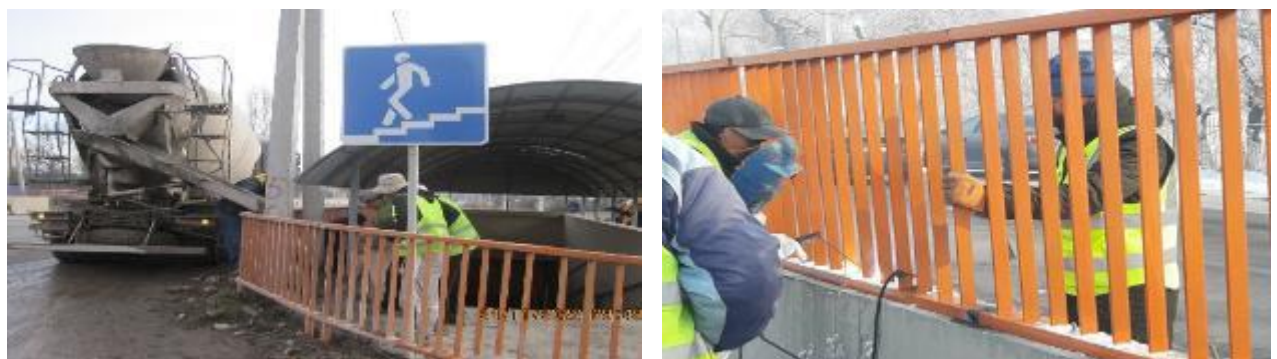
Figure 33 Installation of metal grating in road construction sites
