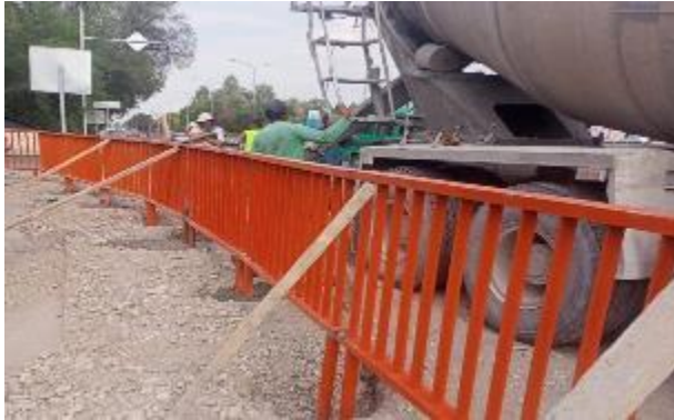
Figure 20 Installation of metal guardrails
