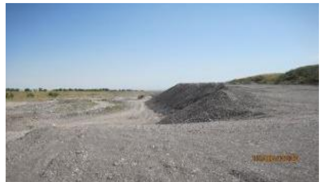
Figure 14 Development of Ak-Suu 2 borrow pit on moistened material
