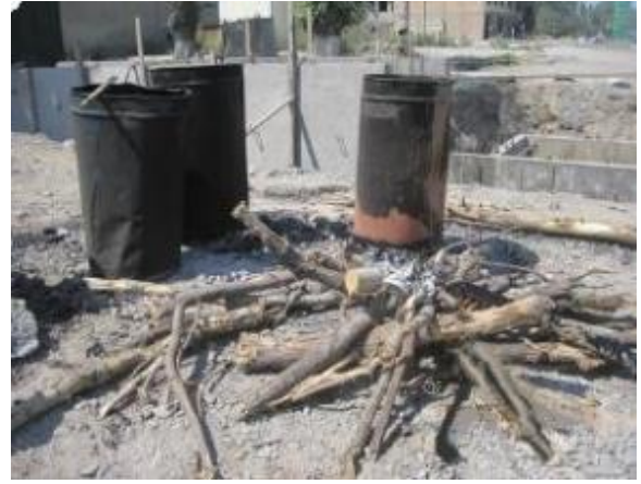
Figure 25 Bitumen melting for waterproofing of pipe
