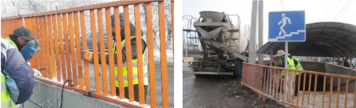
Figure 36 Installation of metal guardrails near underpasses and in crowded places
