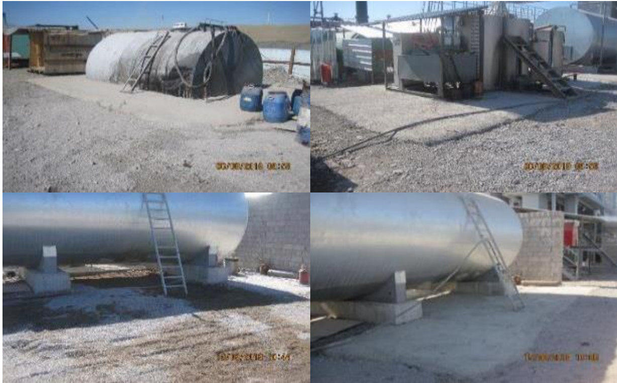
Figure 47 Impenetrable protective coating around chemical containers
