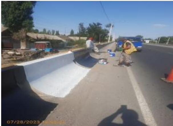
Figure 9 Painting parapets and curbstones
