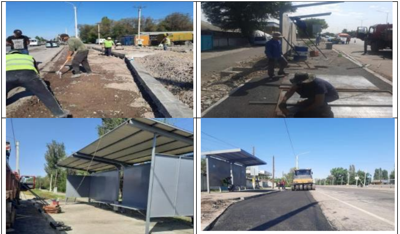
Figure 34 Construction of bus stops
